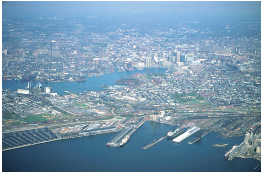
Fig. 2.15 Baltimore Harbor in Maryland has been transformed from a natural harbor at the fall line of the Patuxent River into a major port observed here in 1977, hard armored to stabilize its shore for concentrated development that the city supports today. Photograph © Ray & McCormick-Ray.
